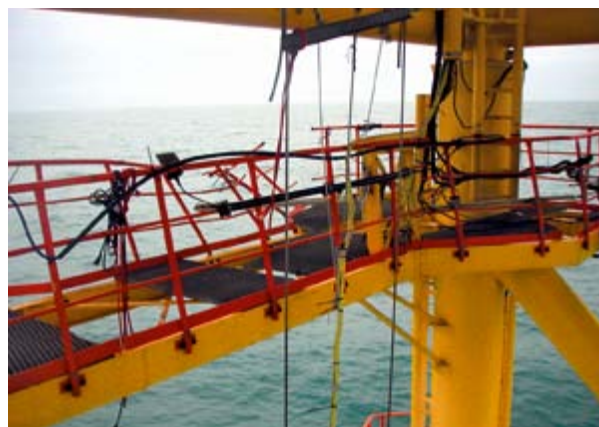
Fig. 2: Results of wave action on the FINO research platform near Borkum
